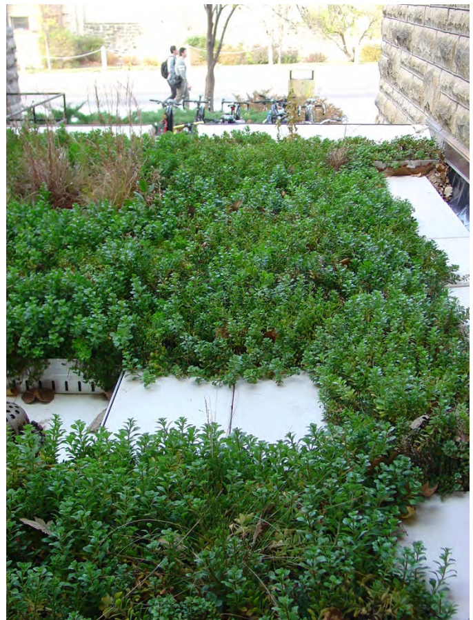
Photo by Lee R. Skabelund – Nov. 9, 2012. Pavers, drain, sedum trays & native plants (going dormant).
