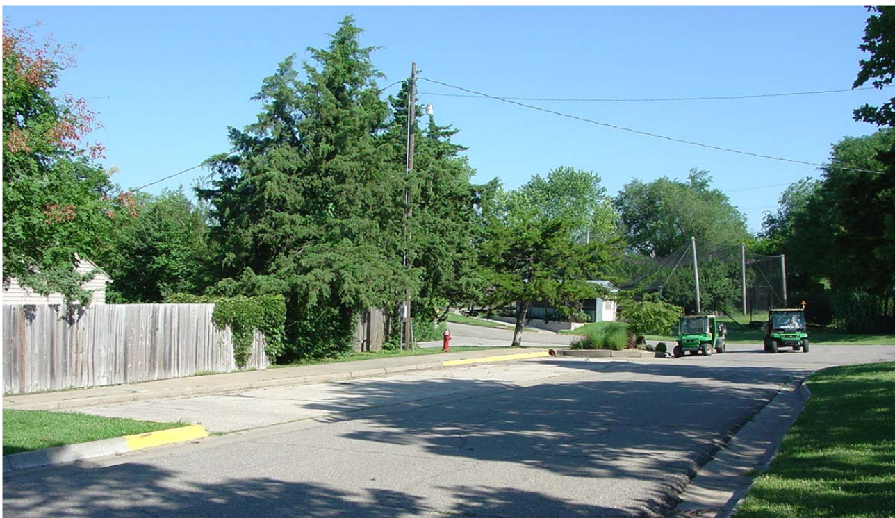
Bio-Retention Area project site prior to construction (underutilized parking area and sidewalk) – July 1, 2010 (Irs)
