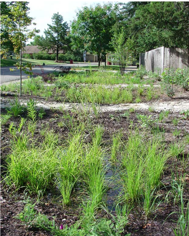
June 21, 2012 photos (lrs) of the pools less than 10 hours after a two-inch, four-hour storm event filled the pools. Infiltration works!
