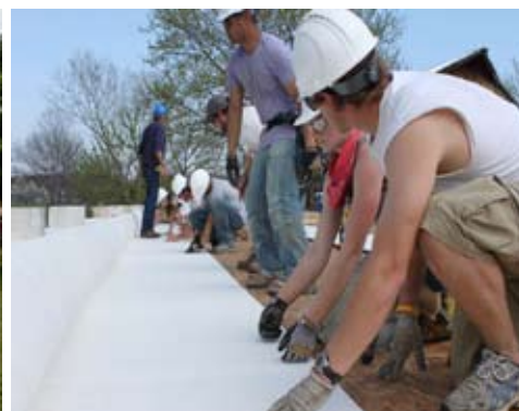
Public Open House - The easily accessible location and high visibility helped shape our choice to use the building to publically demonstrate the latest technologies throughout the design of the building.
