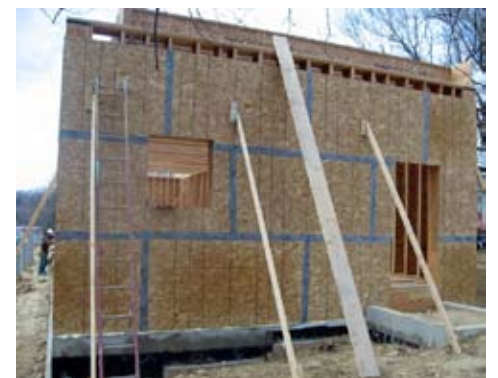
All Construction Joints are Sealed - We spend a great deal of time sealing up the building during the course of construction. All of the joints between materials are caulked, foamed and covered with tape. Air loss at windows and doors has been kept to a minimum by using good installation practices and purchasing the best performing window/frame combinations that are available. We pressurized the building following construction to confirm its tightness and chase down any tiny air leaks that are revealed in the process to seal them up tightly.
