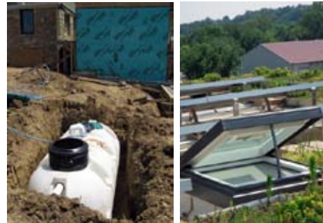
Water Reclamation - Rainwater collected from the roof will be diverted to an underground cistern and used to irrigate the living wall, helping to reduce potable water demands and storm water runoff. It also supplies the toilets.
